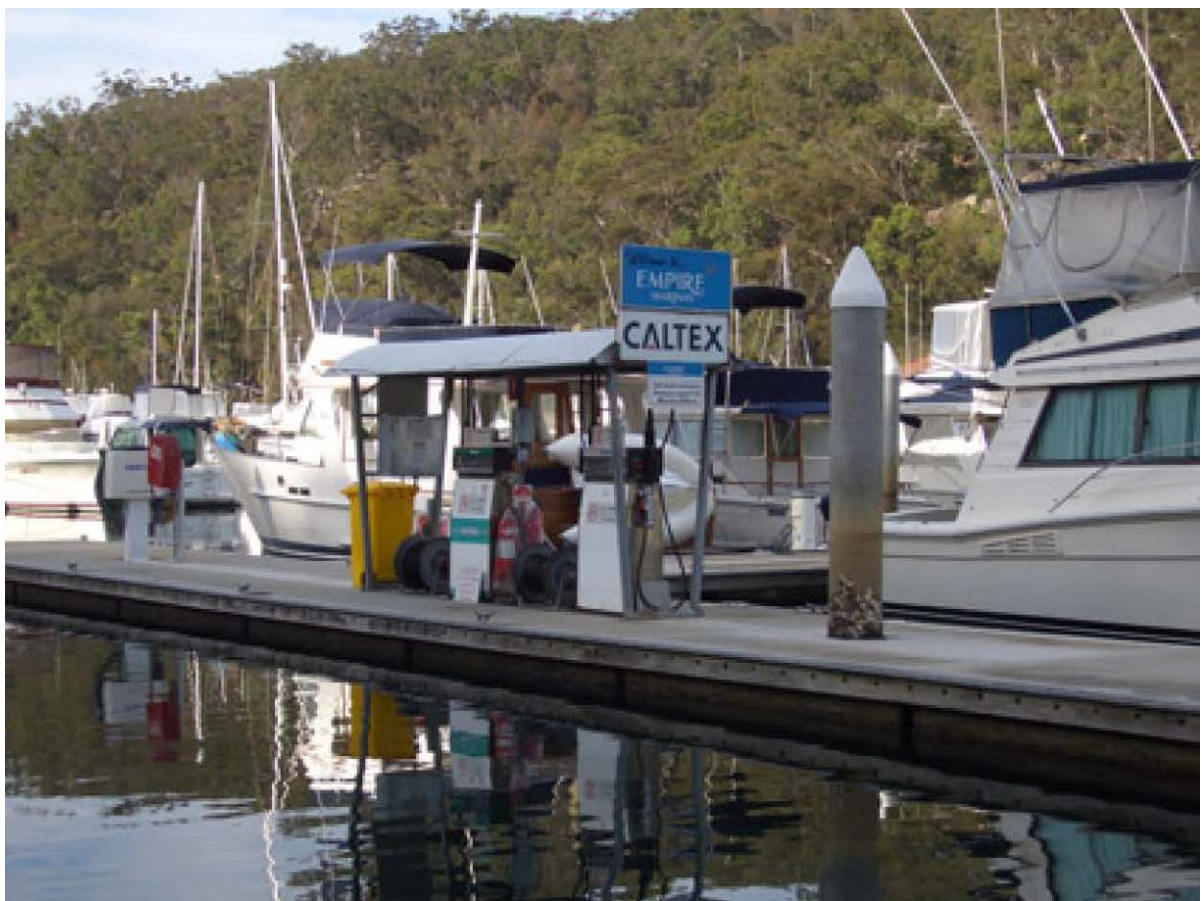
Photograph 2.4 Example of a floating fuel berth (Empire Bay Marina, Bobbin Head)
